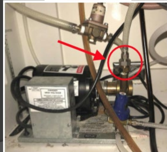
One example of an ASSE Standard 1022 approved backflow prevention device. Devices may vary in appearance. Devices should be labeled ASSE 1022.
